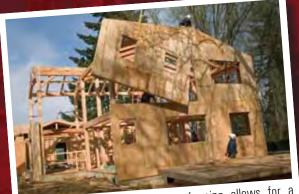
**Enclosing the Frame:** Timber framing allows for a highly efficient home, particularly when enclosed with a pre-cut panel system such as Structural Insulated Panels (SIPs) or our own Matrix wall assembly. Pre-fabricated panel systems provide higher R values and nearly eliminate thermal bridging for optimal temperature regulation, and streamlines time spent on the site.
