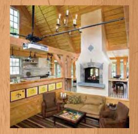
Situated next to the family's in-ground pool and connected to the main home with a timber pergola, this auxiliary timber frame space serves as pool house, guest quarters, and features a golf simulator. Each Douglas fir timber has a custom rough sawn texture achieved through the careful application of a chain saw and wire brushing. Many of the timbers interface with the windows to form a more direct relationship between the structure and the outdoors.
