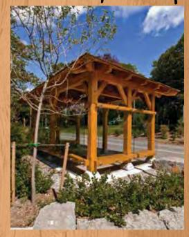
Offering shelter and a place to rest, this 20' x 10' pavilion on Goat Island is the newest in a series of stops for the Niagara Falls Scenic Trolley. The structure is crafted of Douglas fir timbers including benches which serve the dual purpose of adding structural stability and providing seating.
