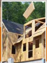
There are other high performance options for the roof and wall system, and we are always trying something new. Whether it's a double wall system that eclipses R-45, 18" deep roof system nearing R-60, or a variety of cutting edge smart membranes, we like to push the envelope (pun intended). Help us understand your goals, and we'll design and build a solution.
